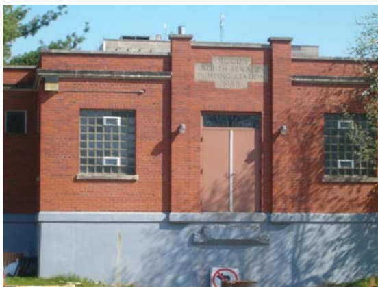
North Side Pump Station
