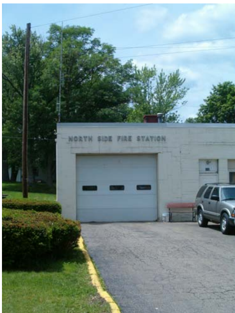
North Side Fire Station
