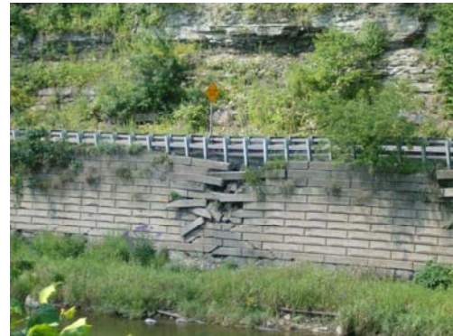
Route 8 Bypass Wall
