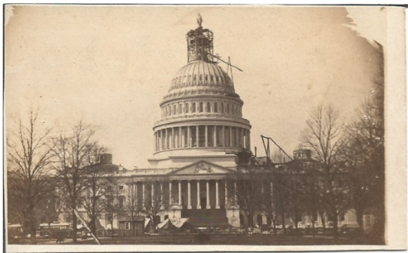
A View of the US Capitol Building Under Construction
