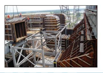
SEI teamed with Sargent and Lundy on Ameren's Coffeen Unit 2 precipitator project. This was a \$12 million engineer, fabricate and supply project for the ESP and associated ductwork. SEI designed and executed a Physical Flow Model of the ductwork from the air pre-heater to the ESP inlet. SEI also designed the duct supports, access walkways and foundations. This project included 611 tons of ductwork and 275 tons of structural steel.
