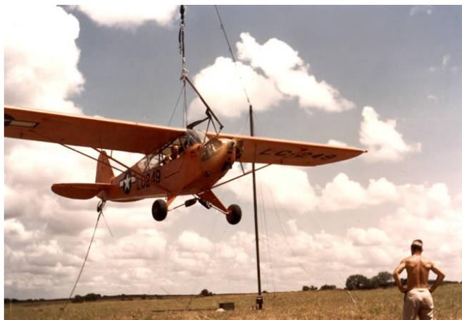
*In this picture, a Piper L-4, engine running, is ready for take-off while suspended from its cable.*
