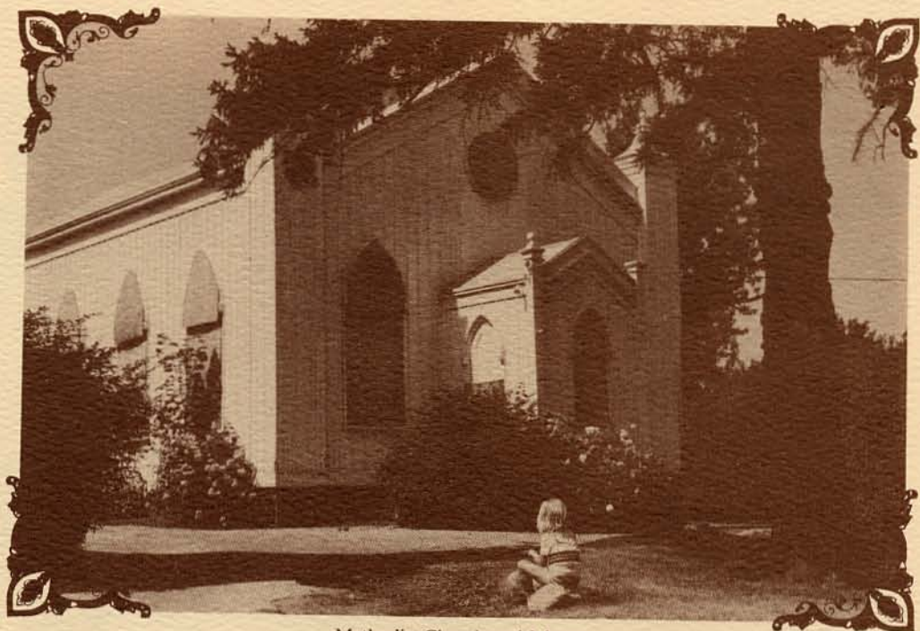
Methodist Church parish house.
