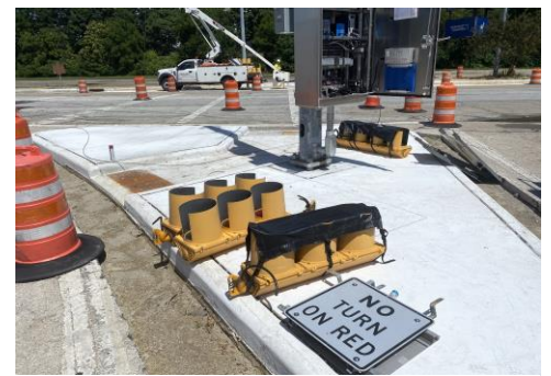
A view from the street of the construction
