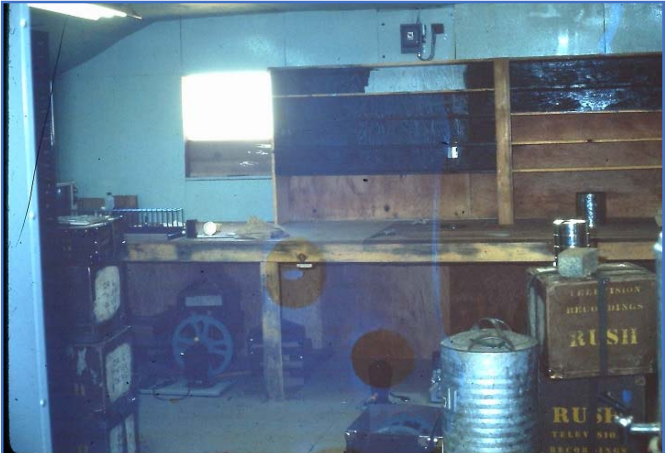
The Production Area Under Construction.
