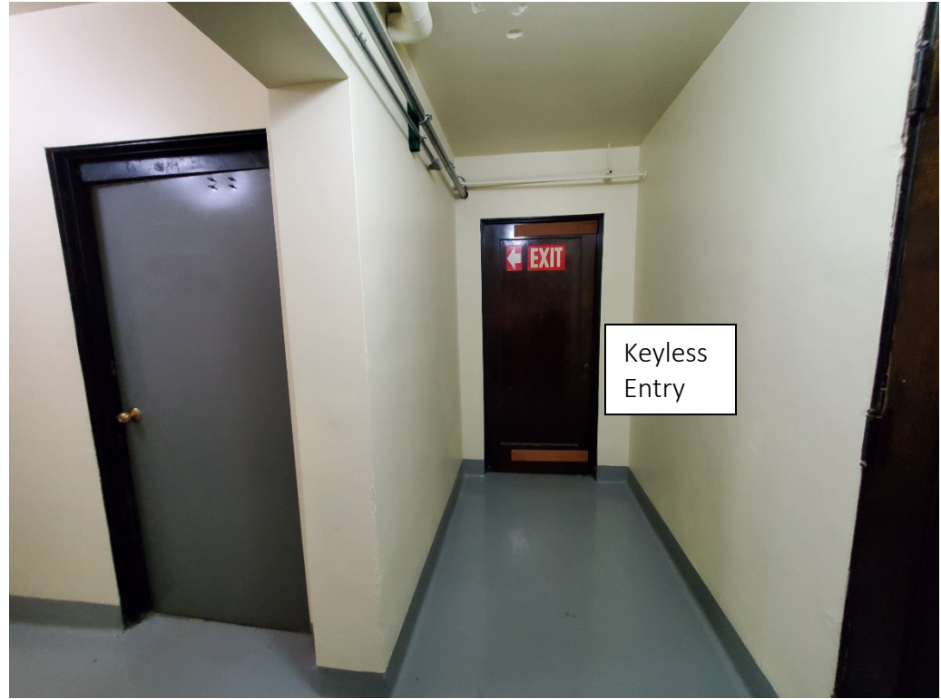
Door 5 Interior IT Room
