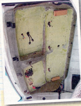
18. The audio components and peripherals were dismounted and the overhead electronics console was mounted into the vehicle. The power connections were made (without fuses, of course) and the console is shown ready to accept the components.
