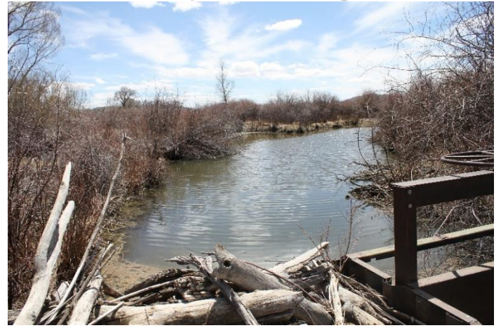
Ditch upstream of headgate
