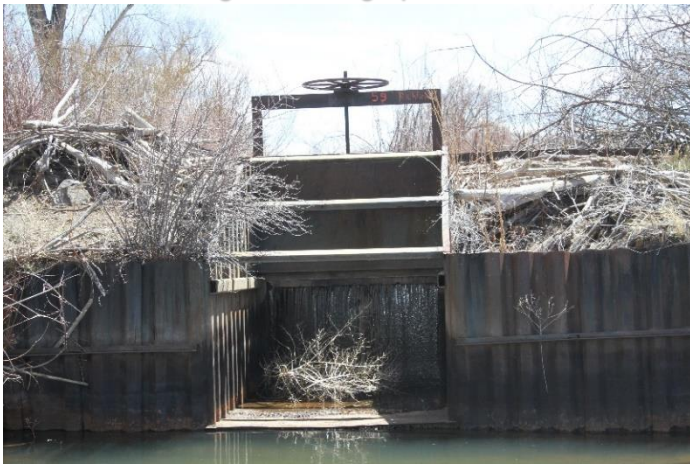
Headgate looking upstream
