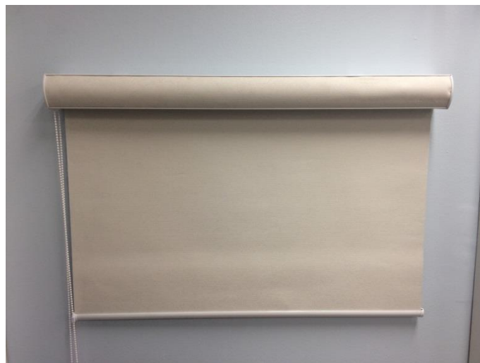
Installed Shade: Outside Mount
