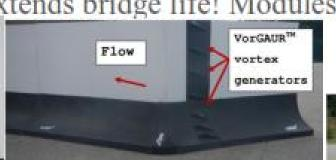
Example stainless steel scAUR<sup>TM</sup> retrofit (black) for a 45° wingwall abutment. Note SS vortex generators.
