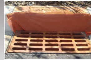
Combination inlet with magnetic rear guard attachment
