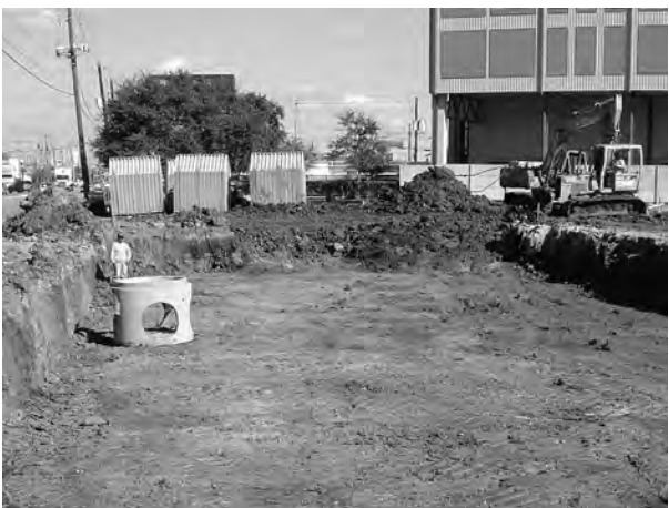
Excavate bed and prepare subgrade per engineer's plans.
