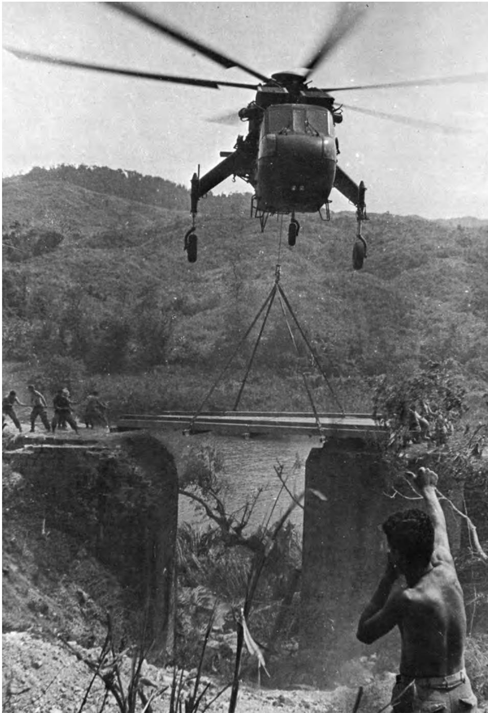
*An Army CH-54 Flying Crane lowers a dry span bridge over a gap as the Marine 11th Engineer Battalion worked to reopen Highway 9 to Khe Sanh during Operation PEGASUS.*
