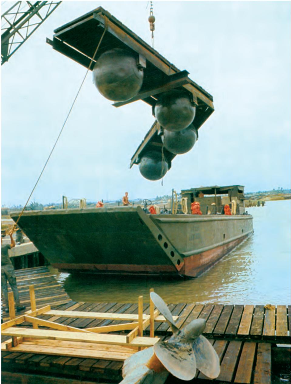
*Floating balls being readied for installation at the Phu Cuong Bridge pier protection system*
