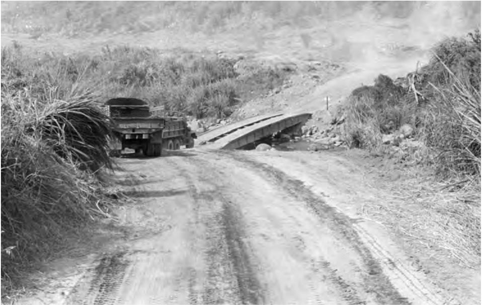
*An armored vehicle launched bridge at Bridge 33*
