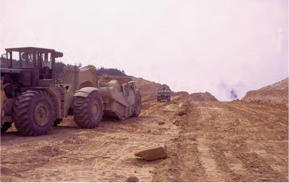
*At the top of Hai Van Pass, the 35th Engineer Battalion deployed equipment like this 290M scraper to widen the road and reduce sharp curves.*
