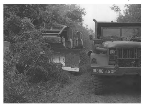
A dump truck and Rome plow begin clearing and widening Highway 9 during the opening phase of LAM SON 719.
