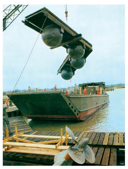
Floating balls being readied for installation at the Phu Cuong Bridge pier protection system
