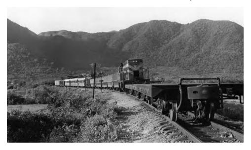
Flatcars on front of a train south of Phu Cat were intended to detonate mines placed on the tracks by the Viet Cong.
