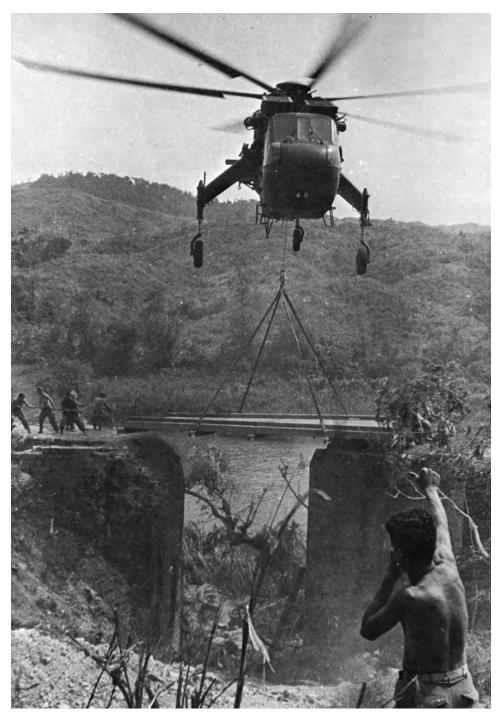
An Army CH-54 Flying Crane lowers a dry span bridge over a gap as the Marine 11th Engineer Battalion worked to reopen Highway 9 to Khe Sanh during Operation PEGASUS.
