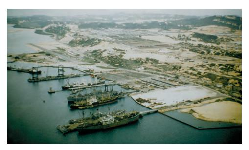
The busy port at Cam Ranh Bay showing a tanker at a petroleum pipeline pier and ships along side of the four cargo piers.
