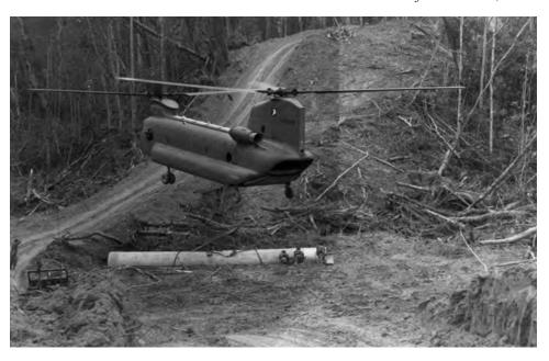
A CH-47 Chinook helicopter drops off preassembled culvert on Route 547.
