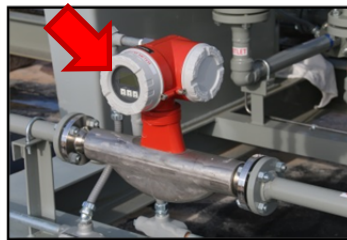
OIL OUTLET CORIOLIS METER FOR MAX. ACCURACY
