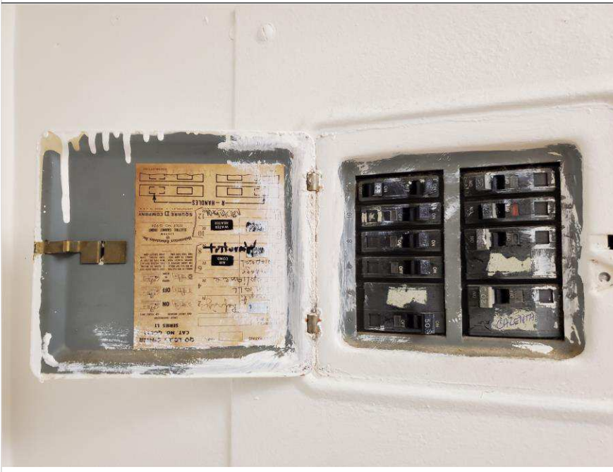
Photo 20 – Village at Dadeland Condominium Association
