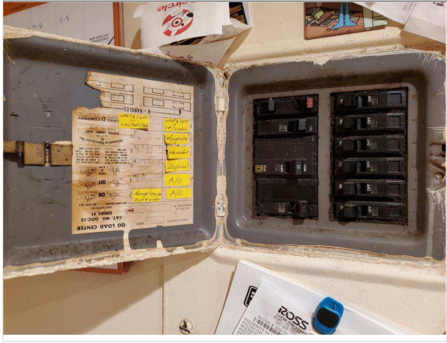
Photo 21 – Village at Dadeland Condominium Association
