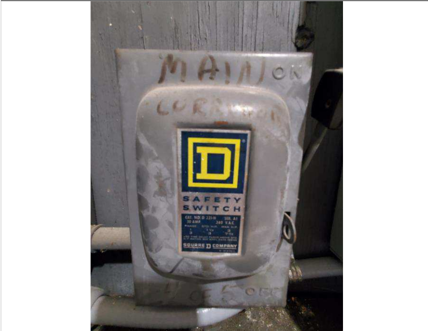
Photo 8 – Village at Dadeland Condominium Association
