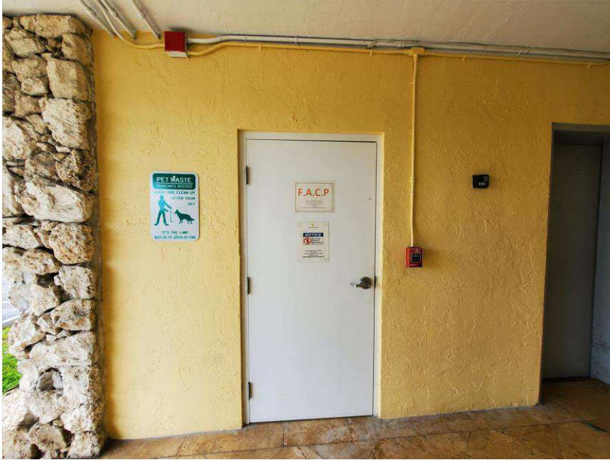
Photo 1 – Village at Dadeland Condominium Association
