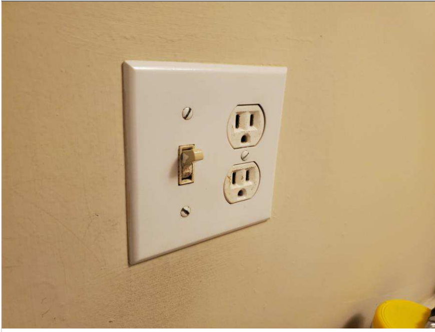
Photo 24 – Village at Dadeland Condominium Association
