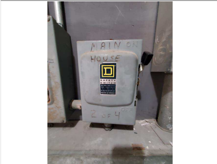
Photo 4 – Village at Dadeland Condominium Association
