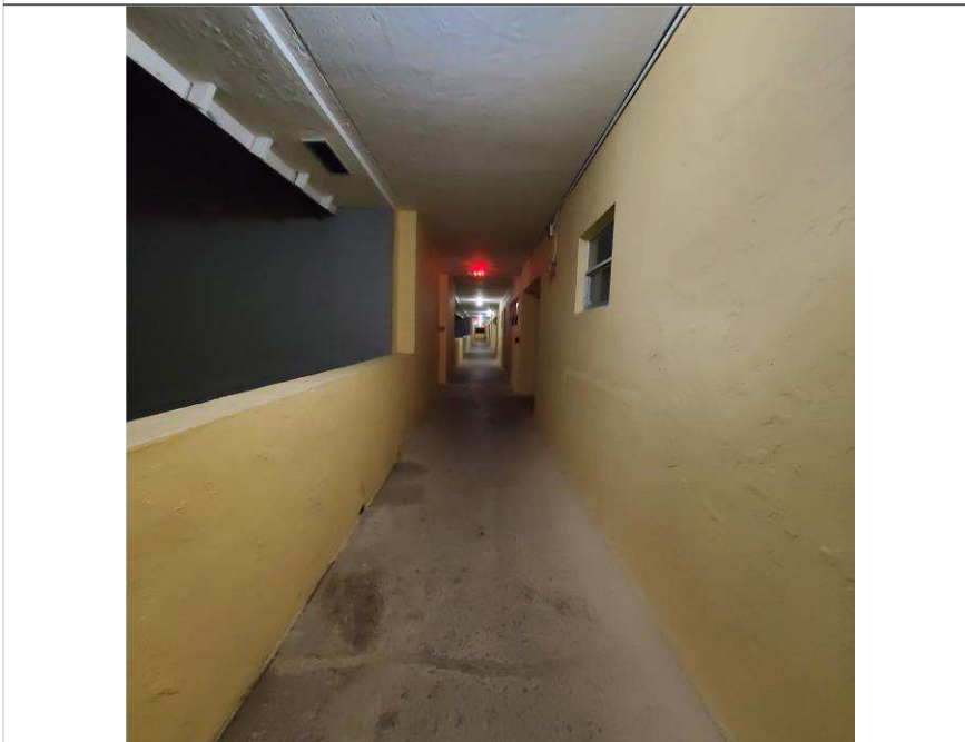
Photo 26 – Village at Dadeland Condominium Association
