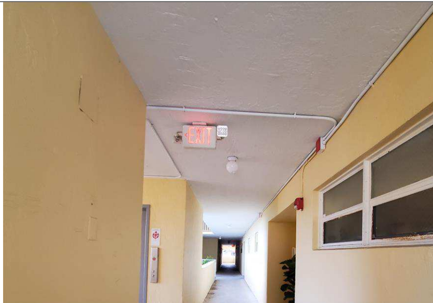
Photo 18 – Village at Dadeland Condominium Association
