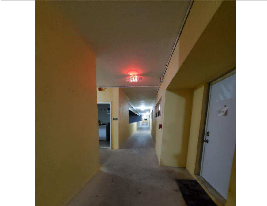
Photo 27 – Village at Dadeland Condominium Association
