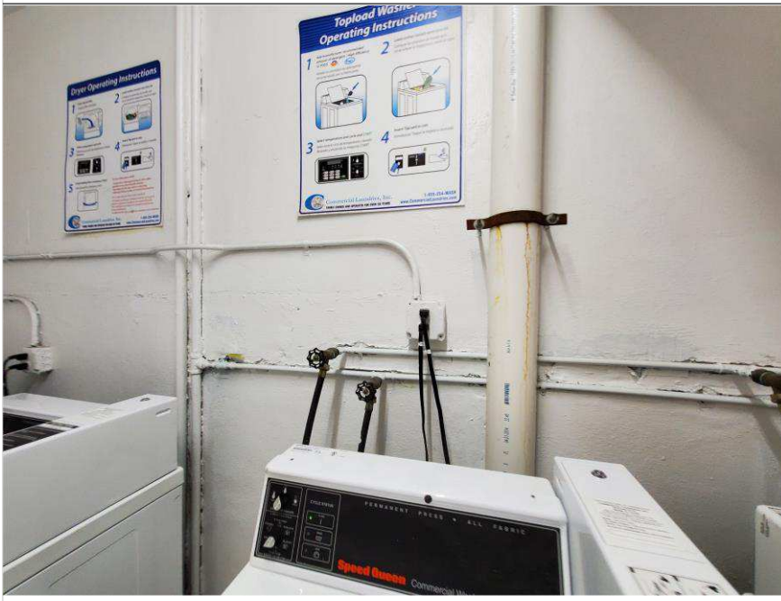
Photo 20 – Village at Dadeland Condominium Association
