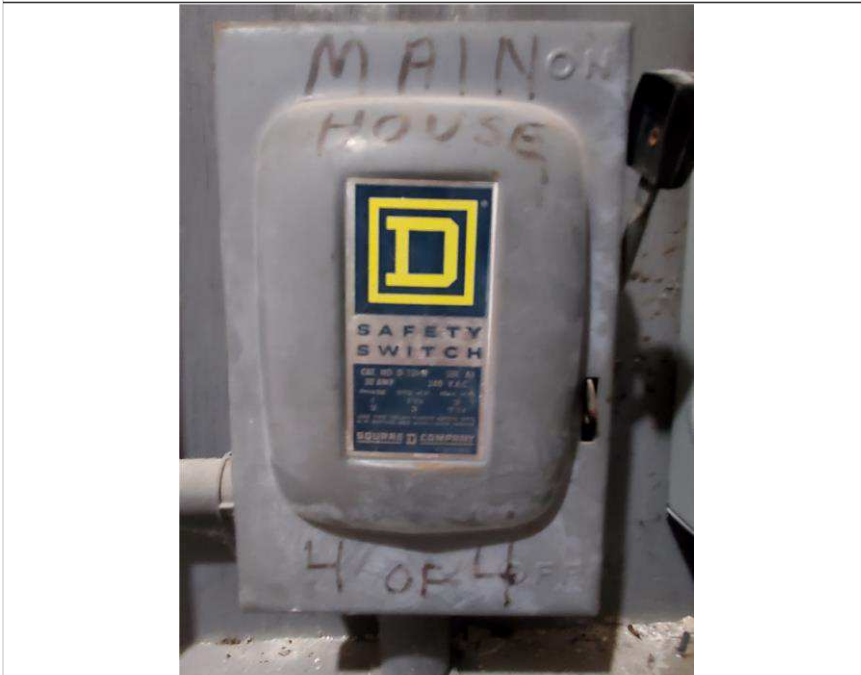
Photo 6 – Village at Dadeland Condominium Association
