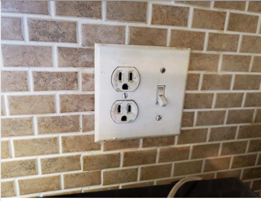
Photo 22 – Village at Dadeland Condominium Association
