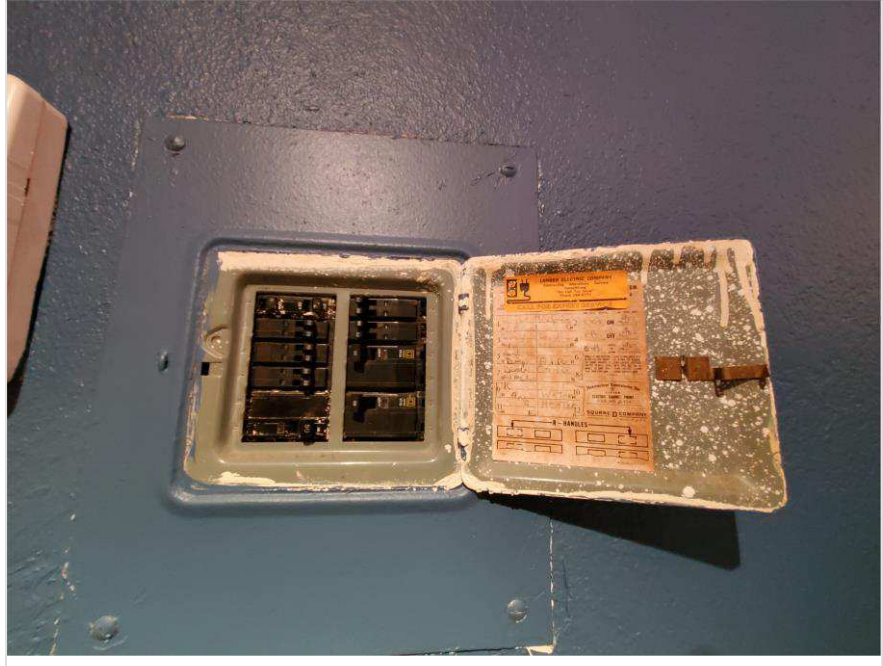
Photo 22 – Village at Dadeland Condominium Association
