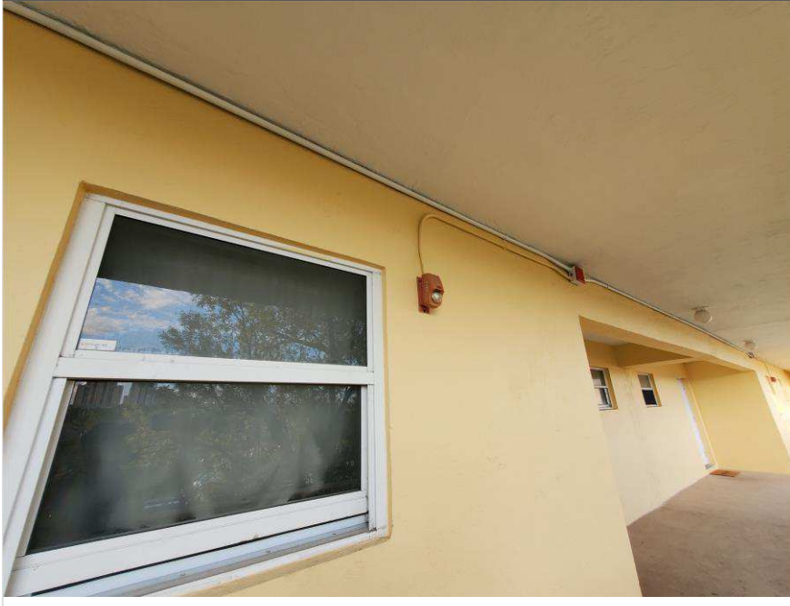
Photo 17 – Village at Dadeland Condominium Association
