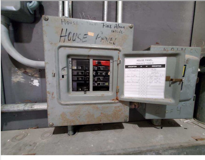
Photo 5 – Village at Dadeland Condominium Association
