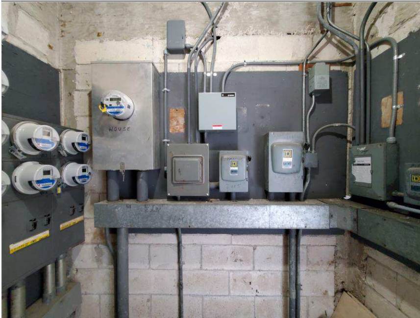
Photo 3 – Village at Dadeland Condominium Association
