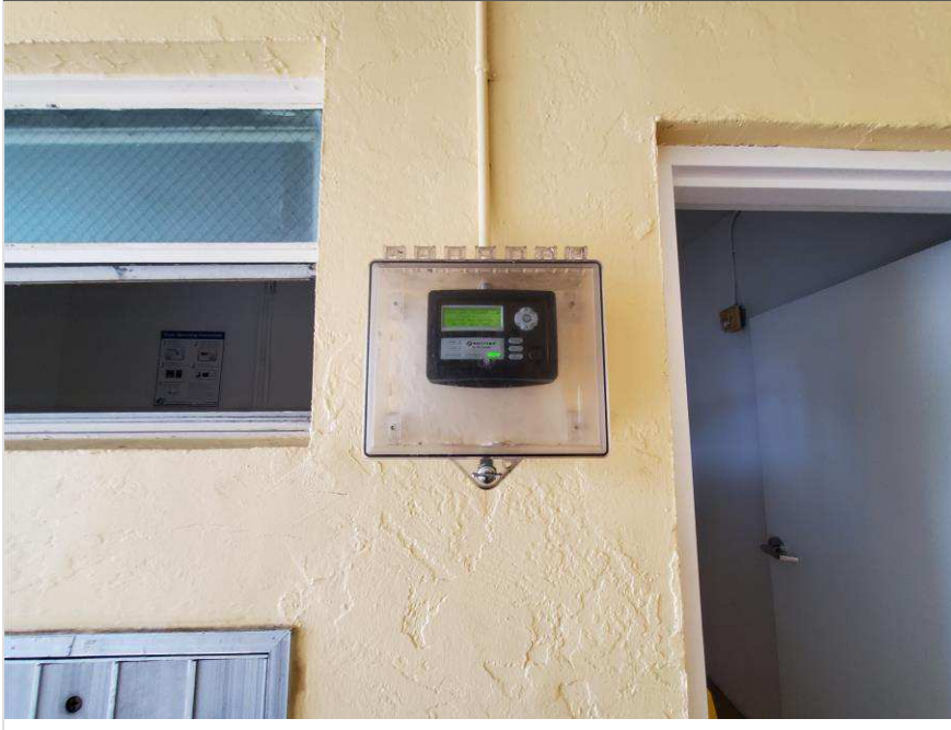
Photo 15 – Village at Dadeland Condominium Association
