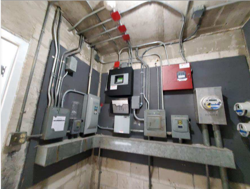
Photo 3 – Village at Dadeland Condominium Association
