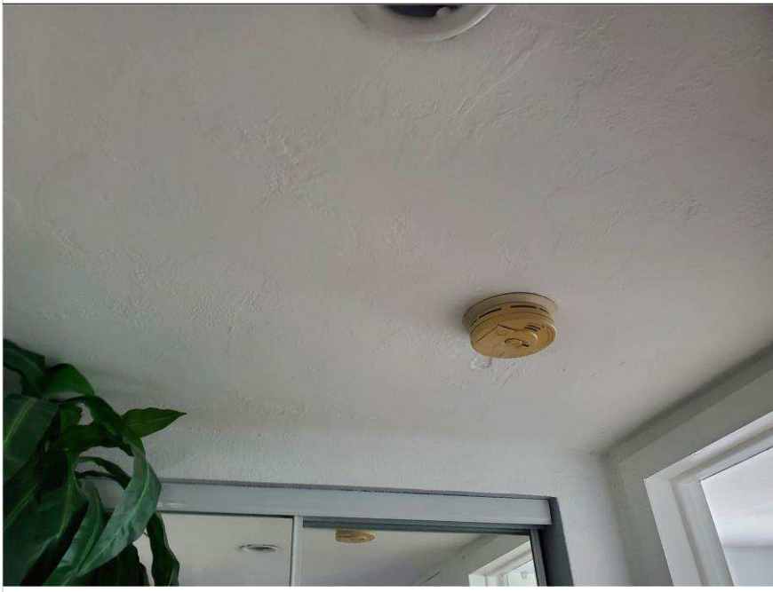
Photo 26 – Village at Dadeland Condominium Association
