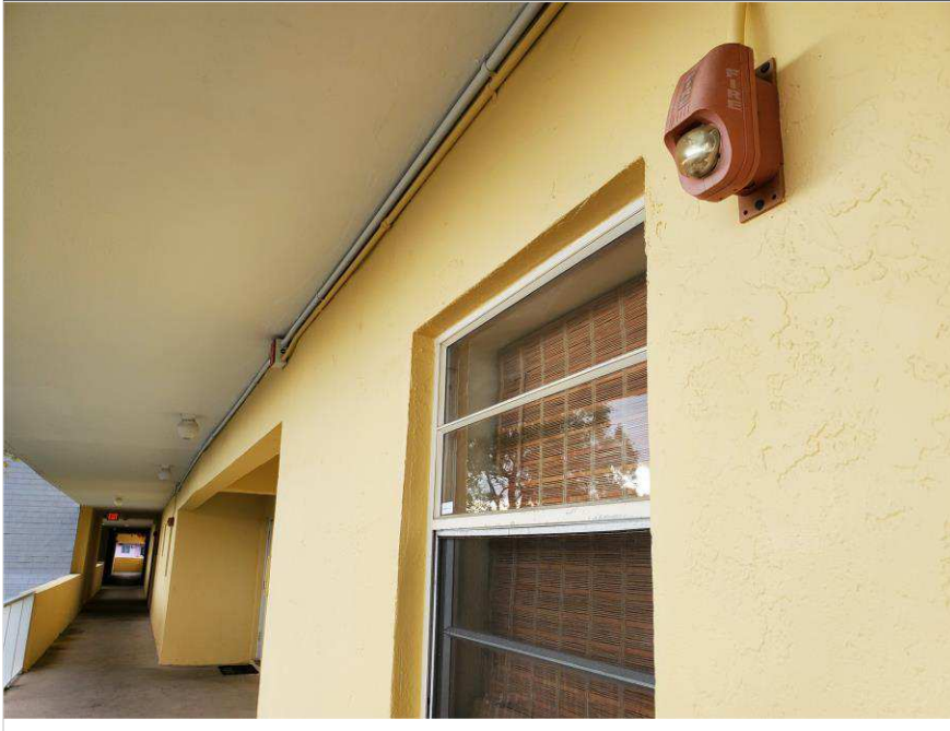
Photo 17 – Village at Dadeland Condominium Association
