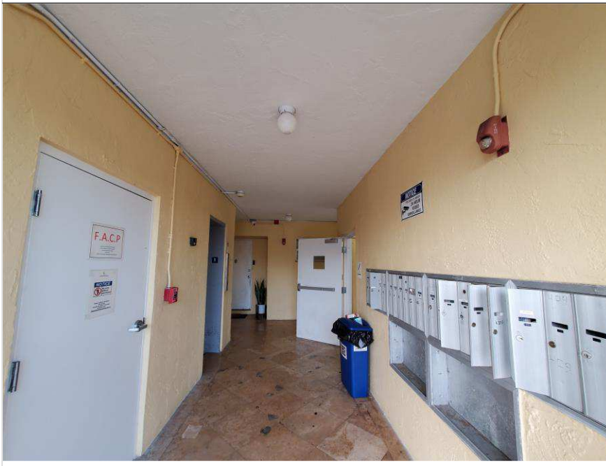
Photo 16 – Village at Dadeland Condominium Association
