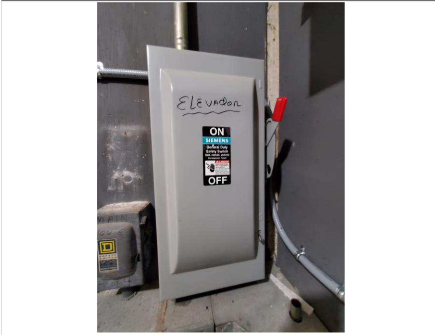
Photo 8 – Village at Dadeland Condominium Association
