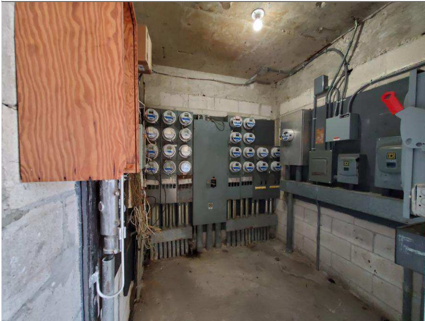
Photo 2 – Village at Dadeland Condominium Association
