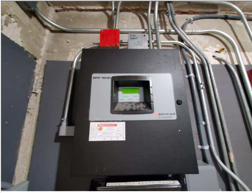
Photo 14 – Village at Dadeland Condominium Association
