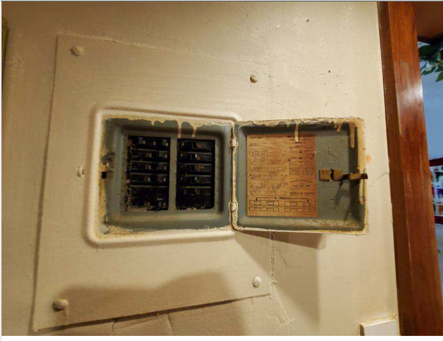
Photo 21 – Village at Dadeland Condominium Association
