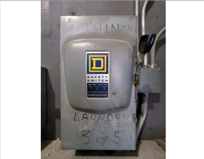
Photo 6 – Village at Dadeland Condominium Association
