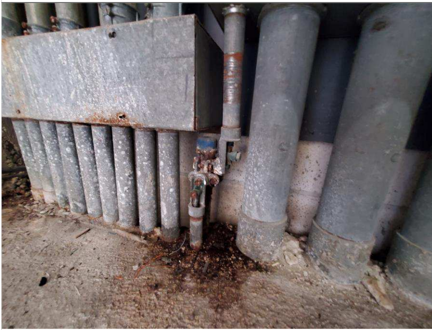
Photo 14 – Village at Dadeland Condominium Association
