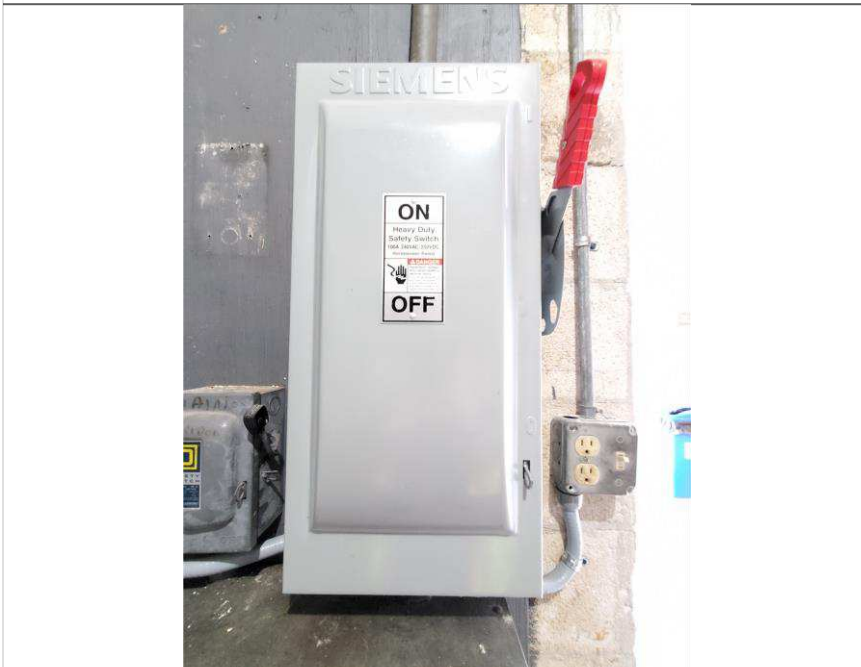
Photo 10 – Village at Dadeland Condominium Association
