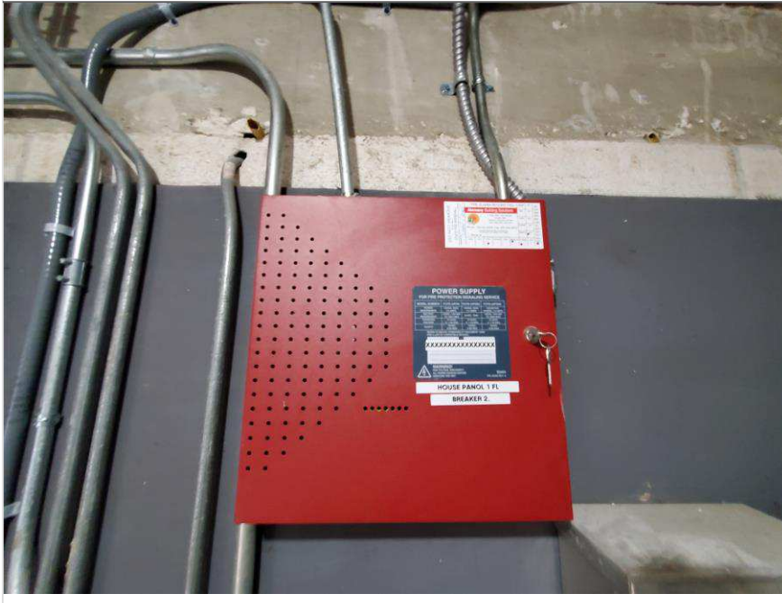
Photo 15 – Village at Dadeland Condominium Association
