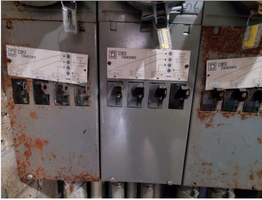
Photo 13 – Village at Dadeland Condominium Association
