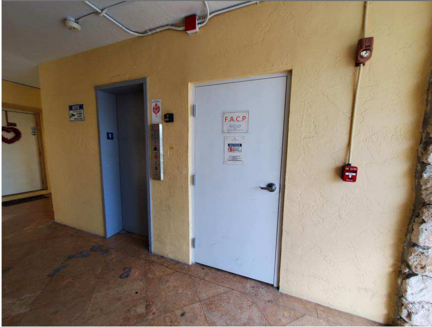
Photo 1 – Village at Dadeland Condominium Association
