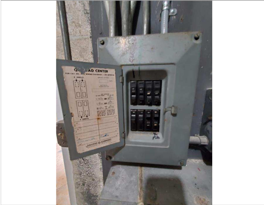
Photo 7 – Village at Dadeland Condominium Association
