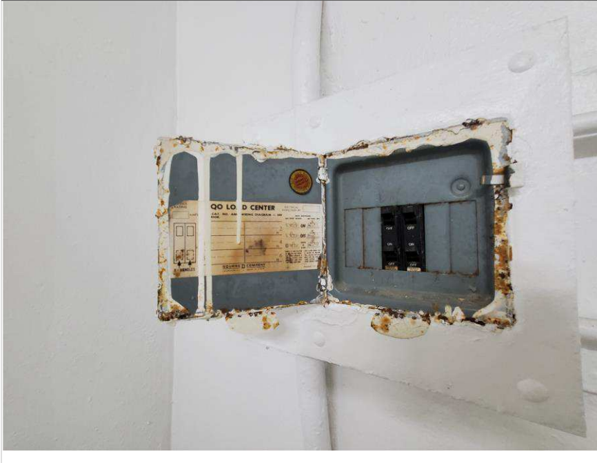
Photo 7 – Village at Dadeland Condominium Association
