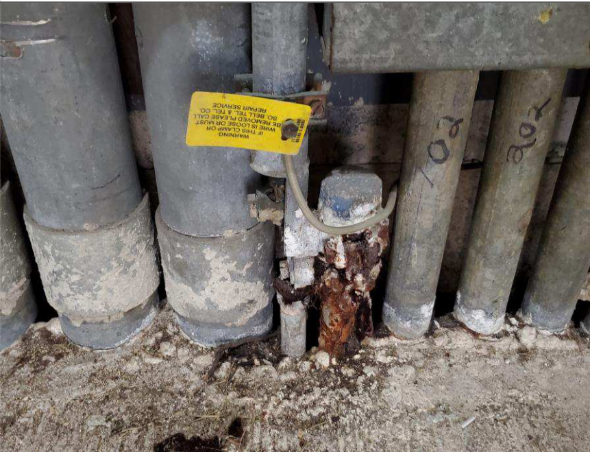
Photo 12 – Village at Dadeland Condominium Association
