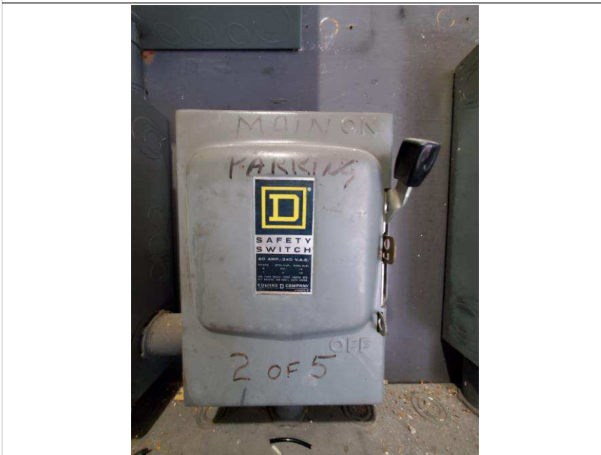
Photo 4 – Village at Dadeland Condominium Association
