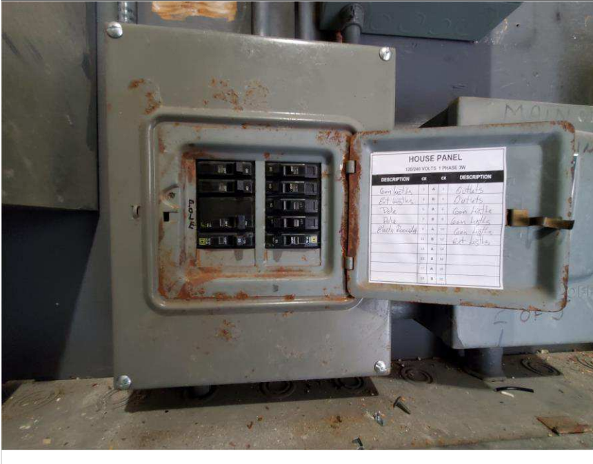
Photo 5 – Village at Dadeland Condominium Association
