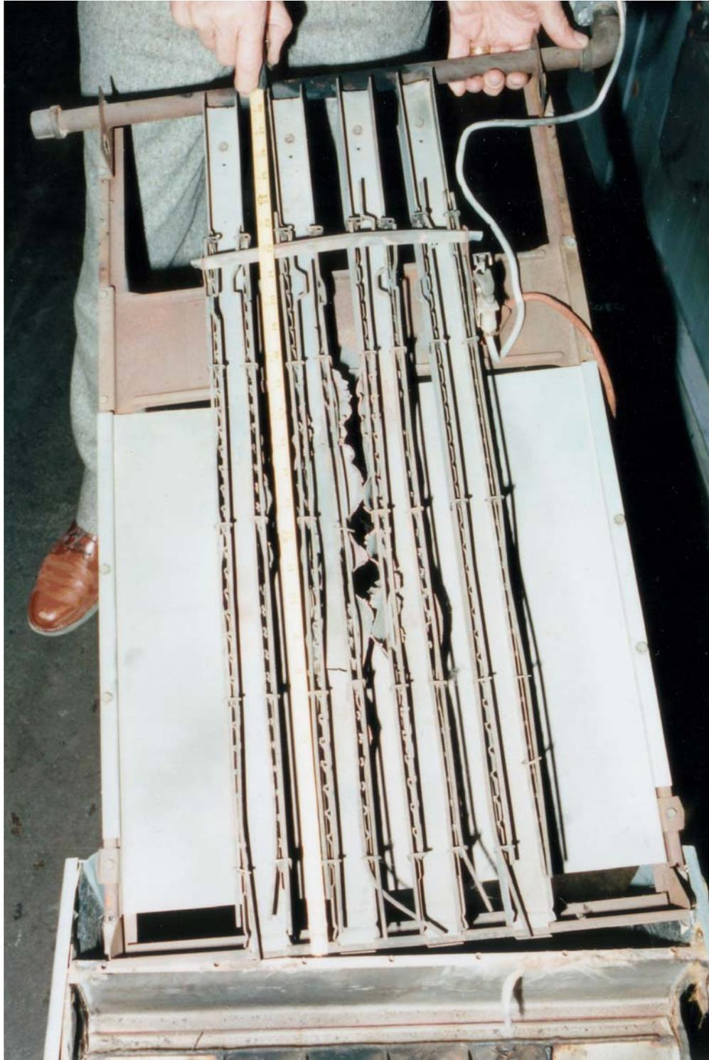
**Photo Five: Damaged burner assembly not equipped with NOX rods.**
