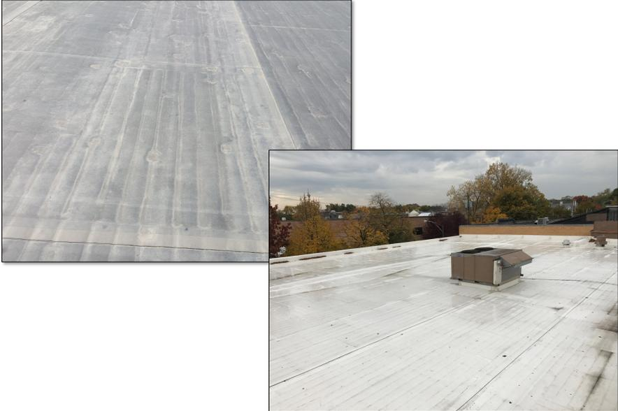
The image contains two photographs. The top-left photograph is a close-up view of a roof surface, showing a grid of lines and circular patterns in the insulation, which are identified as knit lines. The bottom-right photograph is a wider view of a flat roof with a central HVAC unit, showing the same knit line pattern across the entire surface. The sky in the background is overcast.
