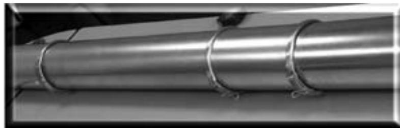
**NOTE: KEEP CUT PIPE IN THE DIRECTION AS THE AIR FLOW.**
