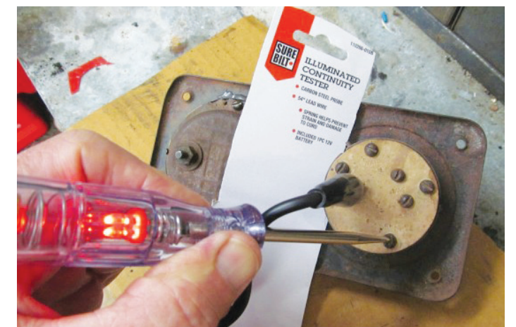
Checking connections on switch plate with a test light
