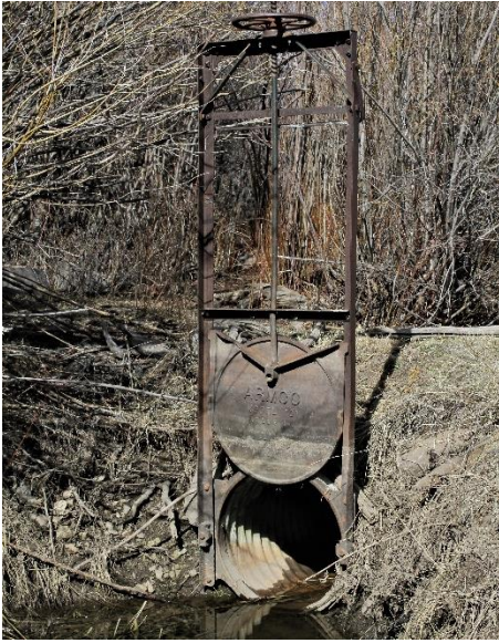
Headgate looking downstream
