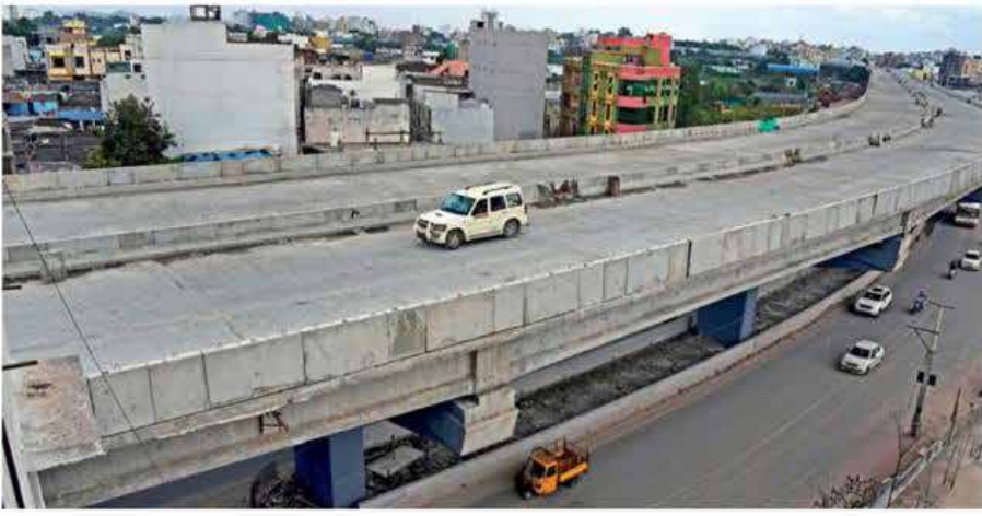
The four km-long flyover from Aramghar to Bahadurpura is on fast pace. The civil works have been completed and it is ready for inauguration —P. SURENDRA
