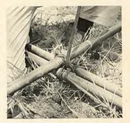
After the three bases are staked, the poles are removed and lashed together at the top with latigo leather straps.
