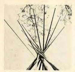
After all but the lifting poles are in place he ties the top together with a half-inch line which goes up on one
