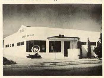
Plant five was built of frame and stucco at 1807 Fifth Avenue, Los Angeles. It was a complete archery shop and at this time Easton further developed his aluminum shafts. Plant was built in 1941 and had 3500 square feet.
