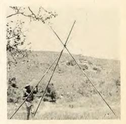
Using the three base poles he lays out an equilateral triangle to position the base of these three poles on the ground.
