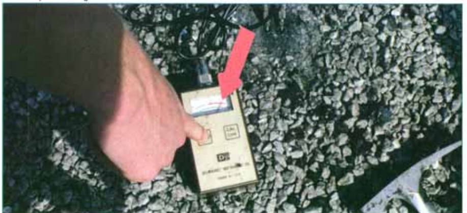
Moisture probe testing of substrate
