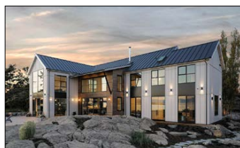
Photo courtesy of Falcon Heights, VRBA's Green Builder of the Year.
