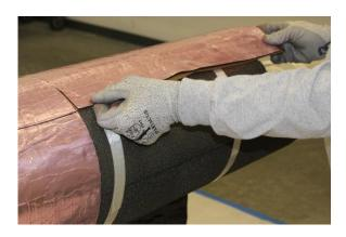
Succeeding sections are applied in the same matter outlined. Succeeding sections are placed to butt against the previous section of jacket. All longitudinal joints should be started on the same line to facilitate placement of butt strips.
