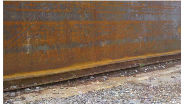
Figure 2 Photo of double bottom with both "chimes" visible
