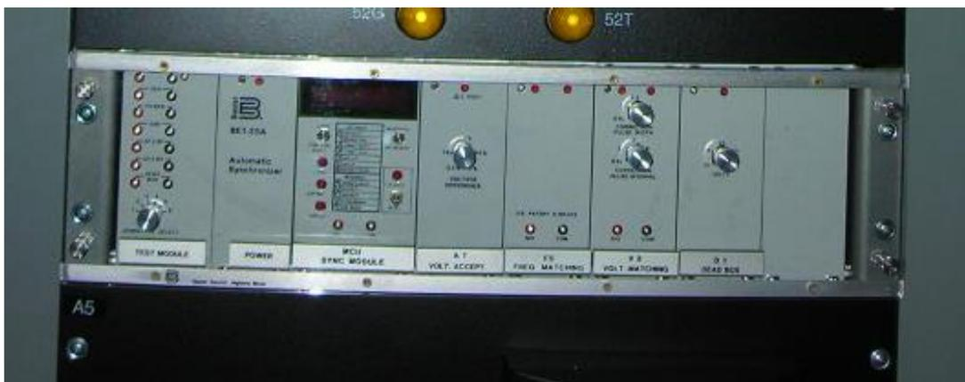
**Current TurboNet *DASH 1*<sup>®</sup> 19" Rack Mount Construction**
