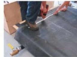
4. EPDM Membrane mechanically fastened with batten bars at the seams
