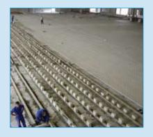
Our capabilities extend from materials supplier to installer. We offer epoxy, vinyl ester, phenol, and furan resins for laying and grouting our proven KNIGHT-WARE<sup>TM</sup> bricks and KNIGHT-GARD<sup>TM</sup> tiles. In addition, our exclusive PYROFLEX<sup>TM</sup> membrane system and sodium silicate cement provides further options for most applications.
