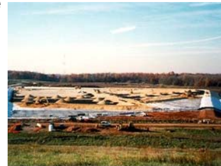
Landfill cell construction, Brown Station Road Sanitary Landfill
