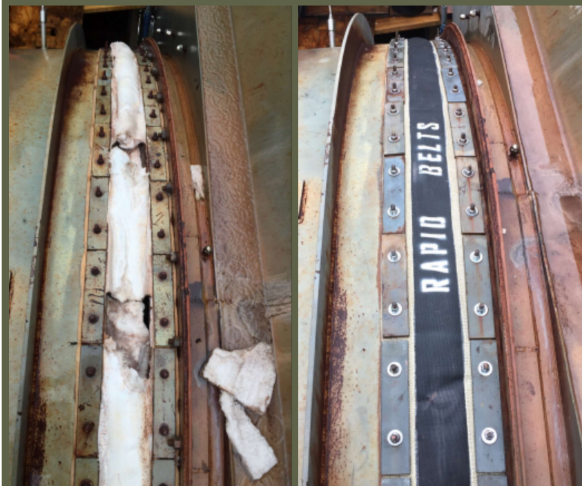
Complete Expansion Joint Upgrades
