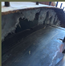
New Upstream Insulation Pack to Replace Missing or Rotten Insulation
