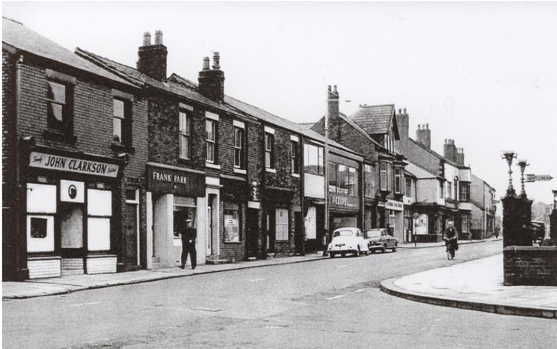
The shop, opposite the Public Hall, in Towngate
