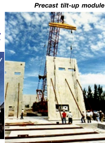
Precast concrete house assembly
