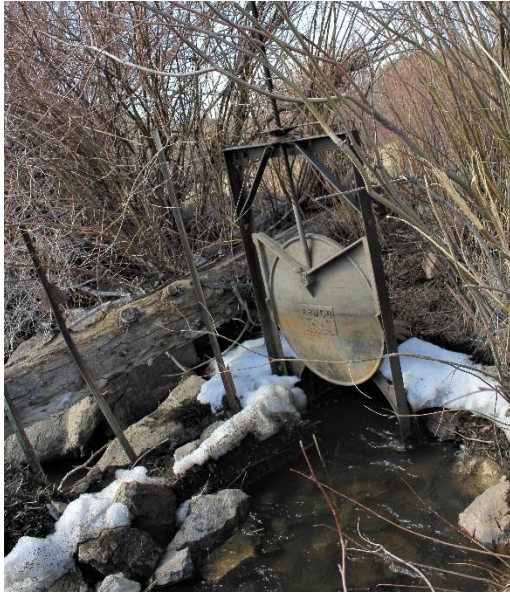
Headgate looking downstream
