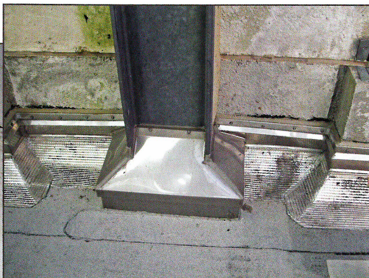
Figure 7 – Sheet metal bonnet installed at I-beam.
