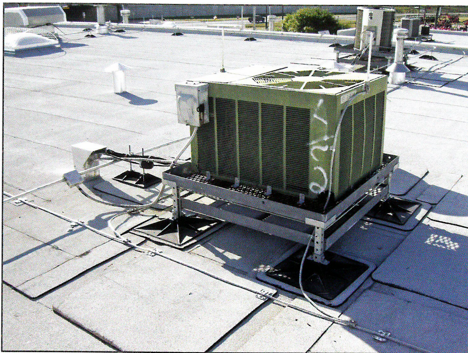
Figure 13 – Mechanical equipment installed on pre-manufactured support.
