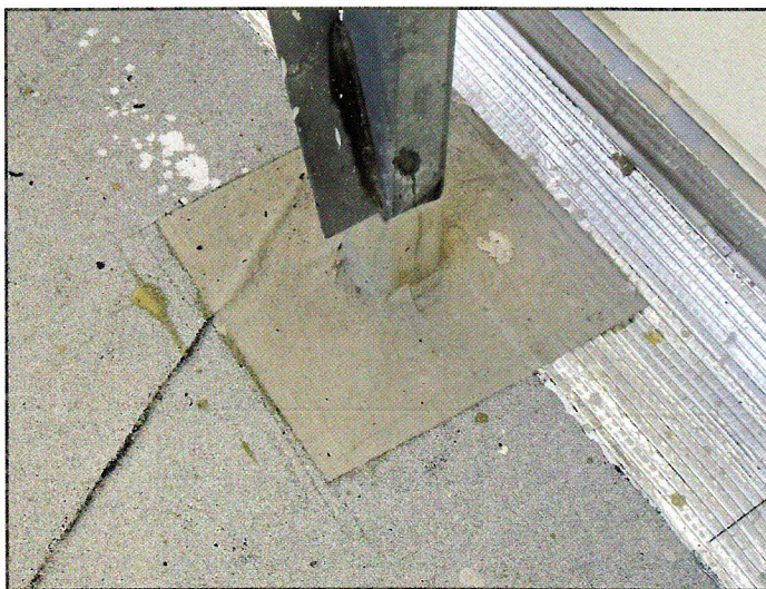
Figure 9 – Liquid flashing membrane installed at steel support.
