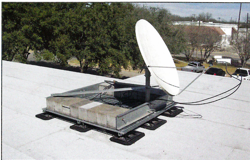
Figure 14 – Satellite dish installed on premanufactured support.
