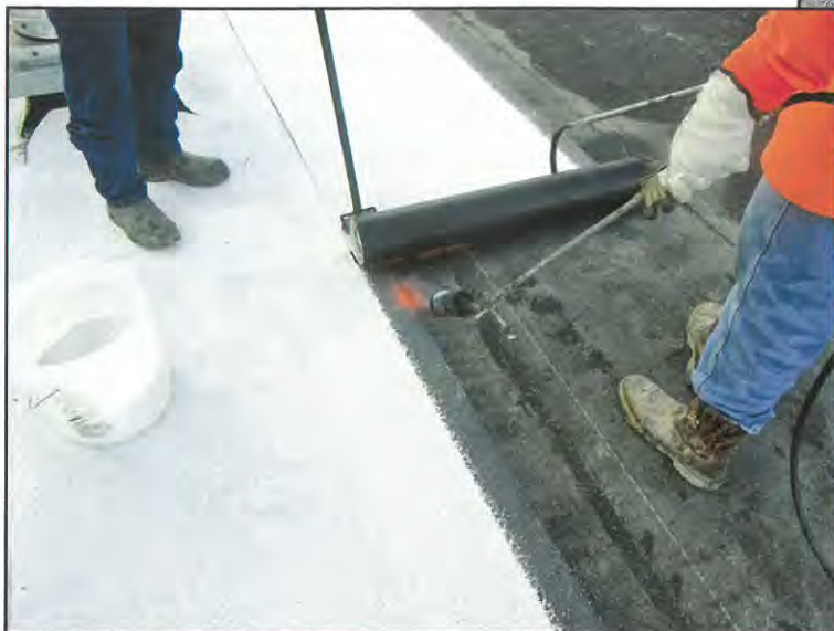
Figure 7 – Torch application of white-colored granule-surfaced cap sheet.
