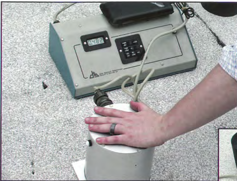
Figure 13 – Reflectivity reading of 48 on cap sheet with stained granules.
