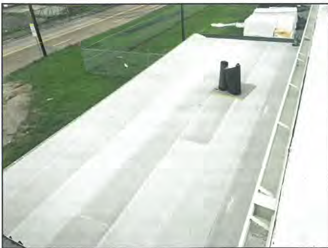
Figure 12 – Varying colors/shades of granules on white-colored granule-surfaced cap sheet.
