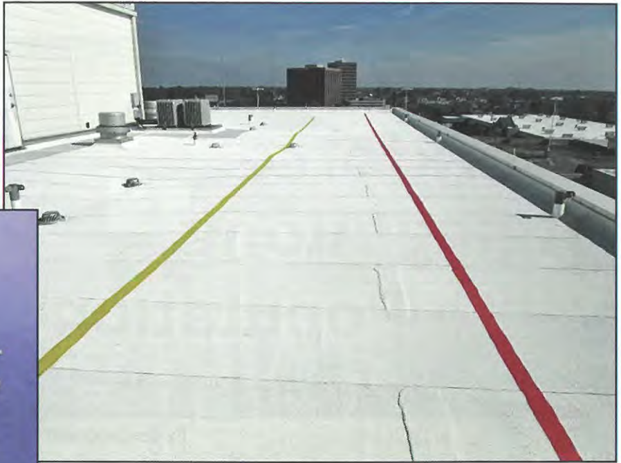
Figure 17 – Overview of installed white-colored granule-surfaced cap sheet.
