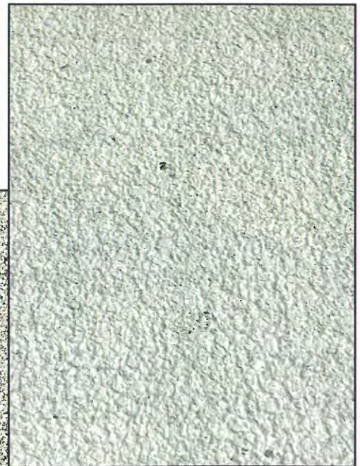
Figure 2 – Close-up of pre-coated granule-surfaced cap sheet.
