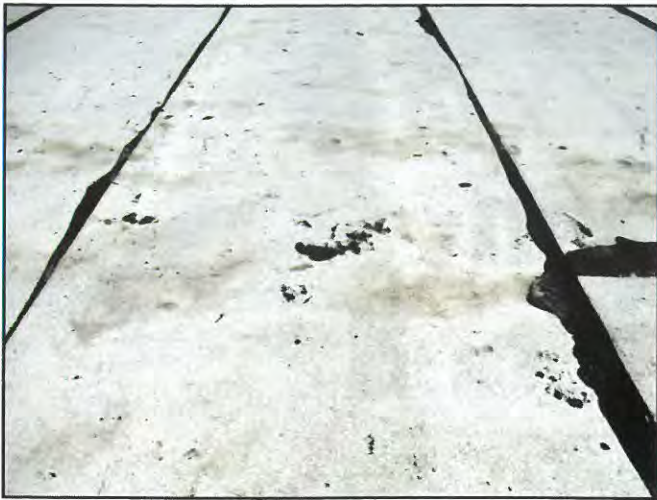
Figure 3 – “Cool” roof cap sheet applied in hot asphalt.
