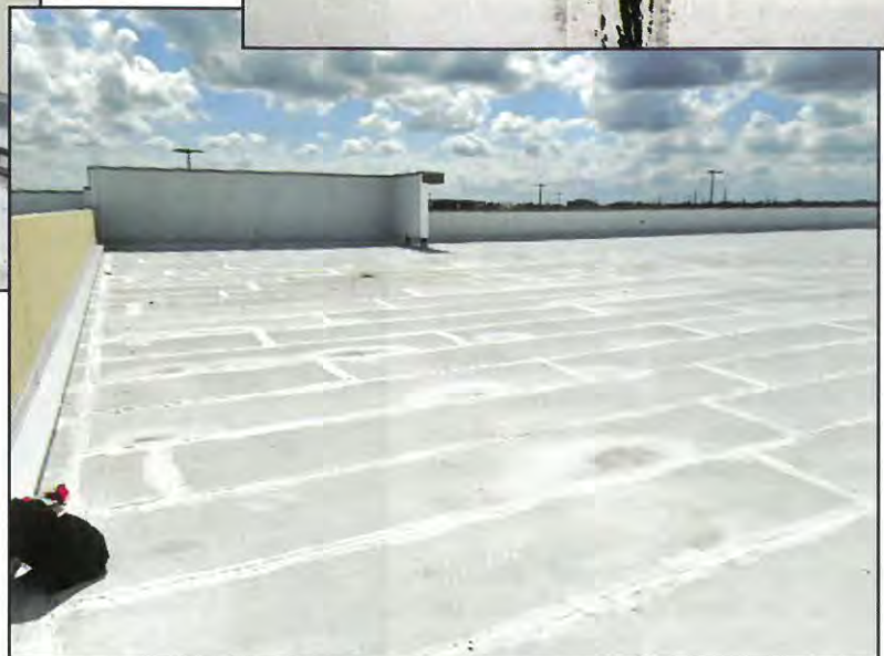
Figure 5 – Bleed-out along laps of cap sheet treated with coating.
