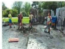
Cleaning up debris from building fire
