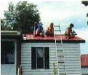
Removing nails from roof, replacing with screws
