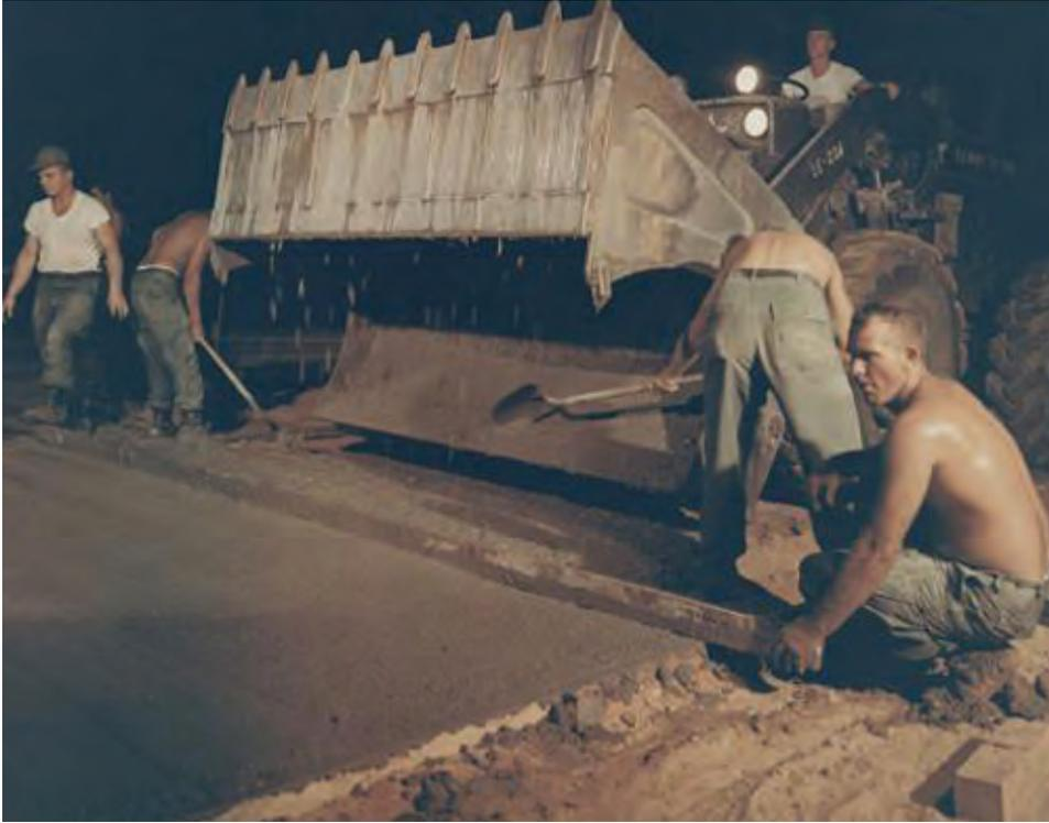
*Because of high daytime temperatures, crews pave concrete pads for buildings at Cam Ranh Bay at night.*
