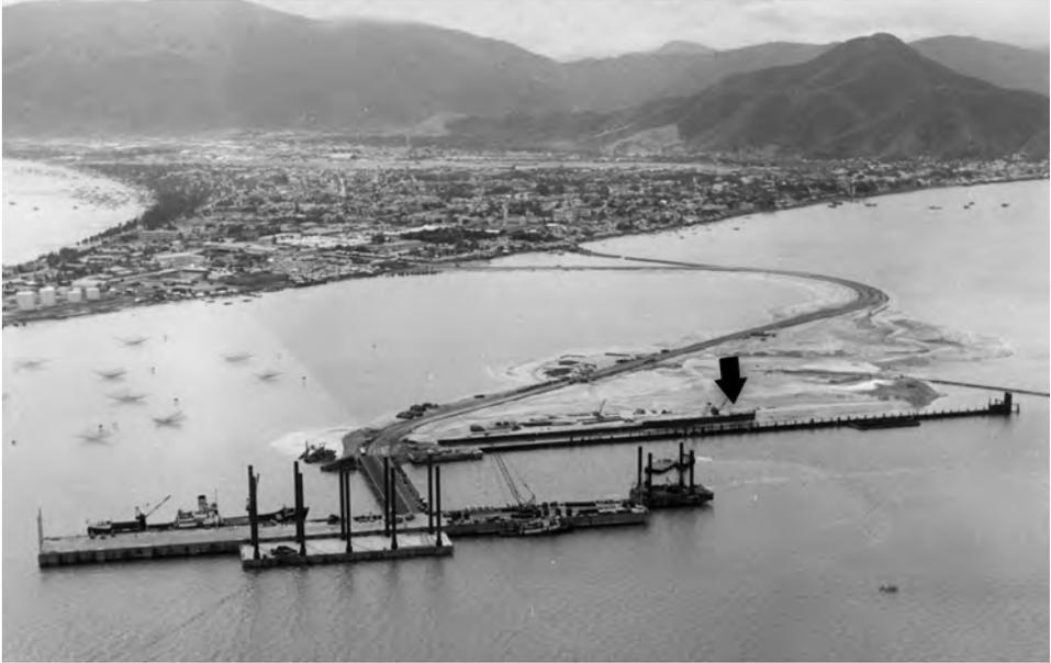
*DeLong pier under construction at Qui Nhon in November 1966. Arrow indicates the hydraulic fill for port hardstand.*
