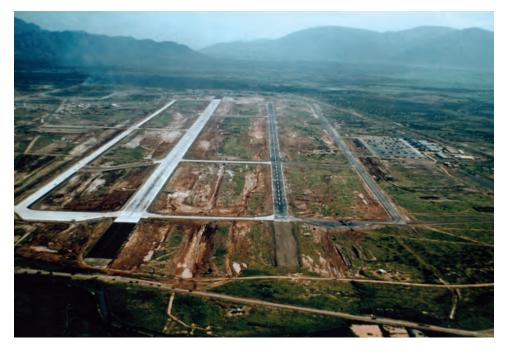
Phan Rang airfield at the end of 1966 showing concrete runway and taxiways on the left and AM2 runway on the right
