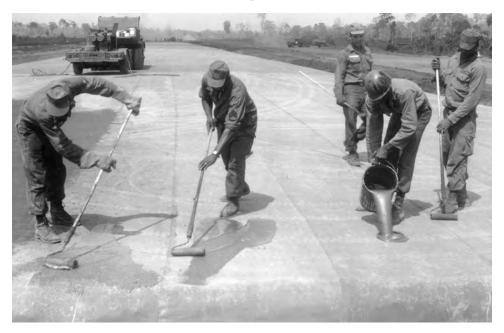
Work crews apply a nonskid compound to Duc Lap airstrip.
