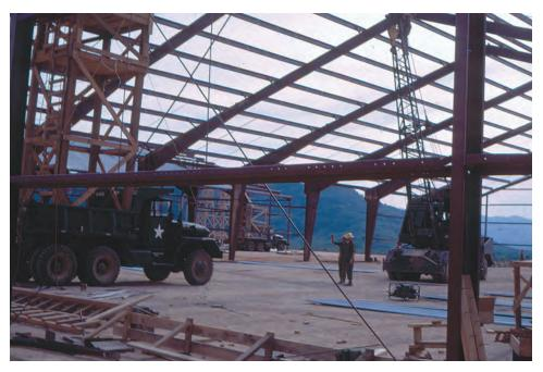
In 1967, construction of depot facilities outside Qui Nhon were under way such as this Butler warehouse building being built by the 19th Engineer Battalion at Long My.
