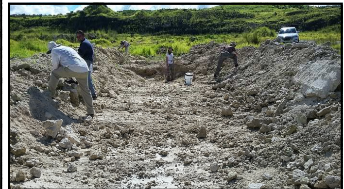
Digging through newly excavated rock
