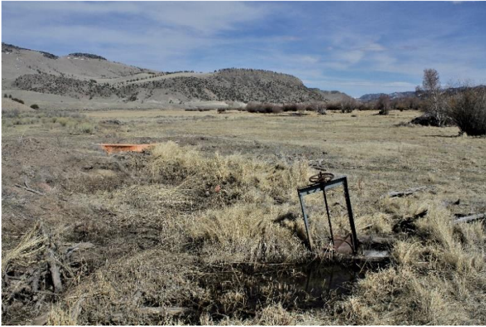
Headgate looking downstream
