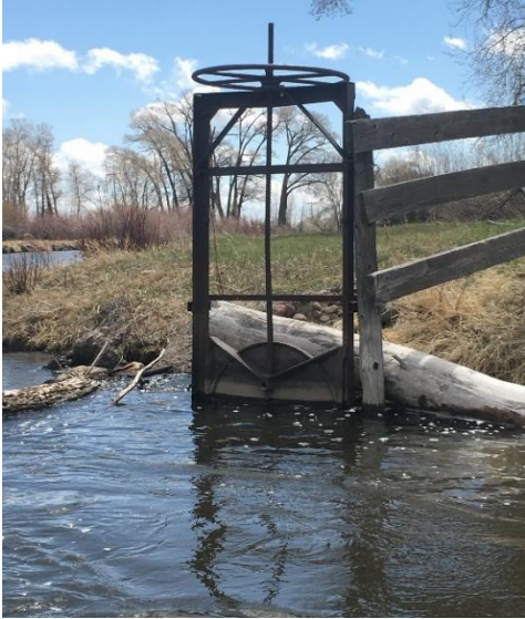
Headgate looking downstream
