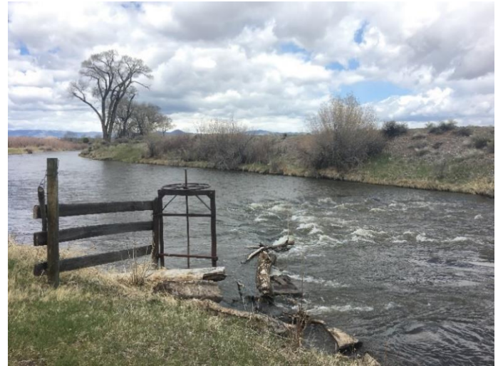
Headgate and diversion dam
