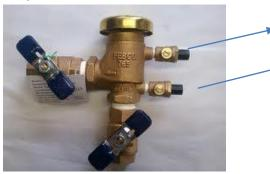
Go to backflow device outside. Turn screws so they are perpendicular to the fitting (up and down).
