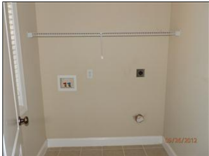
5.15 Picture 1 Laundry Room
