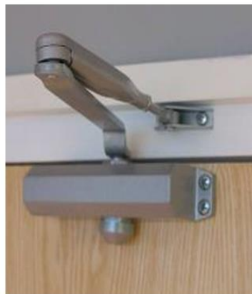
Over-Head Self-Closing Device
