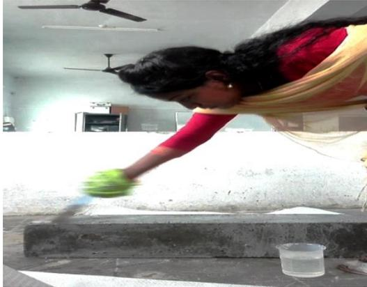
Fig.1: Application of epoxy and hardener on the beam
