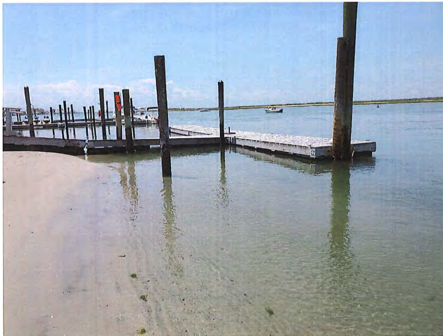
Photo #6: View from the waterline facing west showing the existing docking facility to be removed and proposed dredging area.
