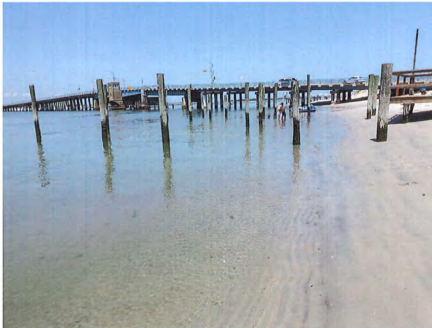
Photo #6: View from the waterline facing west showing the northernmost marina area rendered unusable due to accretion of sand. The existing piling are to be removed and this area is proposed to be renovated as part of the proposed 100% transient marina design.
