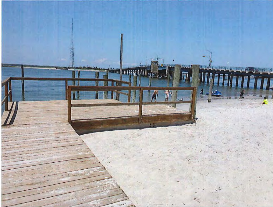
Photo #5: View facing north showing the northernmost fixed pier to be reduced, extended and utilized for ramp access as part of the proposed 100% transient marina design.
