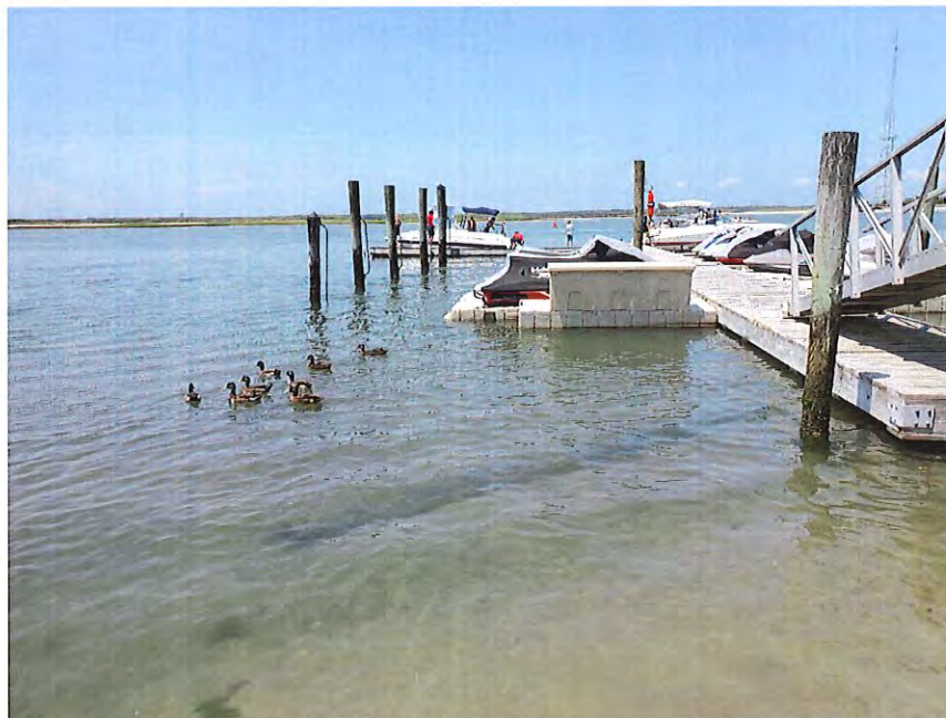
Photo #2: View from the most southerly beach area facing northwest showing "A" dock and accretion of sand requiring dredging.
