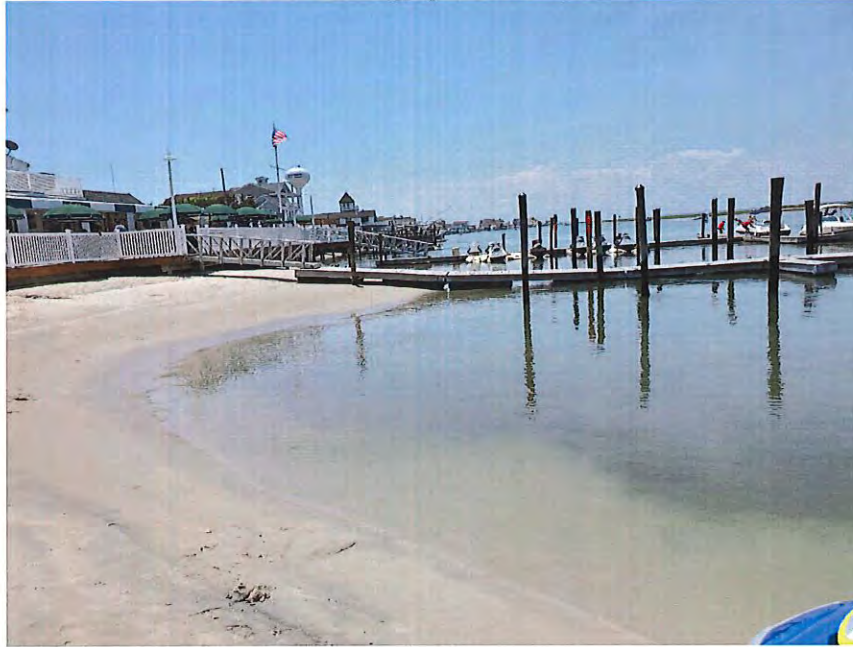
Photo #5: View facing southwest showing the existing “A” and “B” docks to be removed and replaced with a proposed 100% transient marina.
