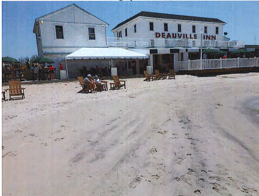
Photo #1: View from the beach showing the existing Deauville Inn Restaurant and Tavern. Notice the accumulation of sand due to seasonal accretion. Areas within the existing marina basin are proposed to be dredged and sand used as beach nourishment for Strathmere Beach as part of Upper Township's Beach Management Plan and Beach and Dune Maintenance Permit
