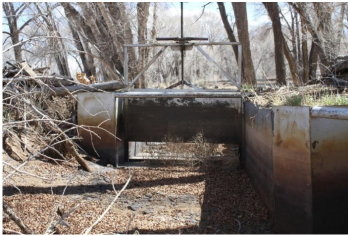
Headgate looking downstream
