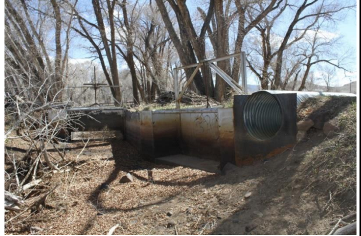
Headgate and diversion dam
